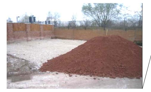
Photographs 9 and <u>10</u>: Inert crushed sandstone being delivered with remediation break layer visible in Photograph 10. The spatial area of the remediation can be observed from these photographs (old terrace housing in Photograph 9 and traffic lights in photograph 10).
