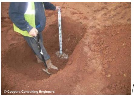
Photographs 11 and 12 show the remediation of the rear garden, with a significant depth (1.0m) of inert cover. Remediation break layer visible at the base of the excavation. Photograph 11 has been stitched to form a panoramic photograph and
